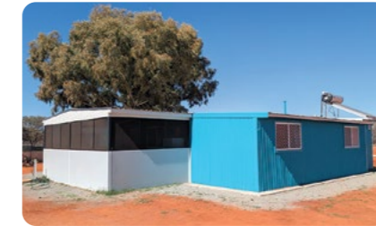
A homelands house refurbished under the HHIP.
